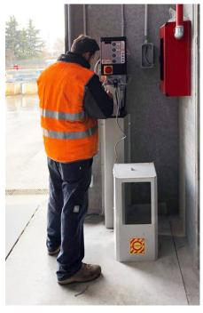
The routine inspection is reduced to the simple oil level check inside the wall positioned CONSOLLE at about 1,5 m H from ground.
